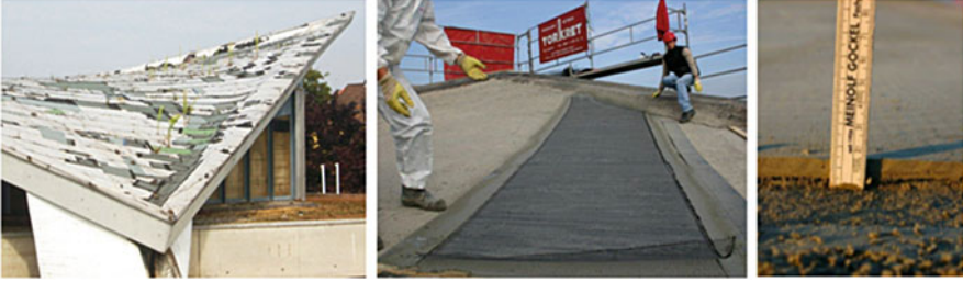
Fig. 16.29 Reinforcement of the hyper shell structure at FH Schweinfurt
