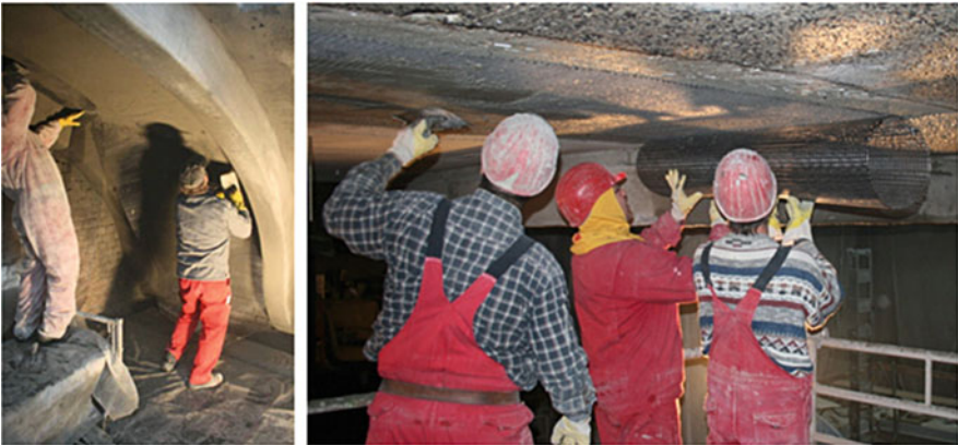
Fig. 16.30 Installation of the textile concrete reinforcement layer
