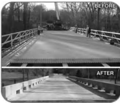
Figure 23.7 GRIDFORM™ FRP reinforcement of concrete bridge deck (prefabricated FRP double-layer grating, concrete-reinforcing system with integral stay-in-place form for vehicular bridge decks) can be seen in the figure [54].
