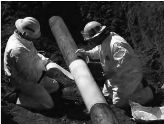
Figure 23.10 Repair of corroded transmission pipeline by wrapping [61].
