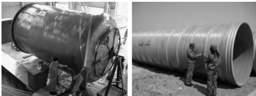
Figure 23.11 FRP vessels and pipes with a diameter of 4–15 m can be repaired by filament winding [63, 64].
