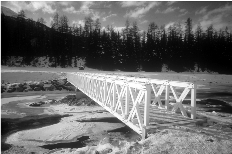
Figure 3.1 Pontresina composite bridge, Switzerland (adhesively-bonded joints connect the glass fiber-reinforced polymer (GFRP) profiles).
