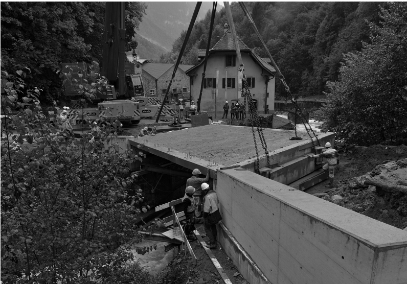
Figure 3.2 Composite bridge deck, Bex, Switzerland (adhesive bonds used to assemble the composite deck).
