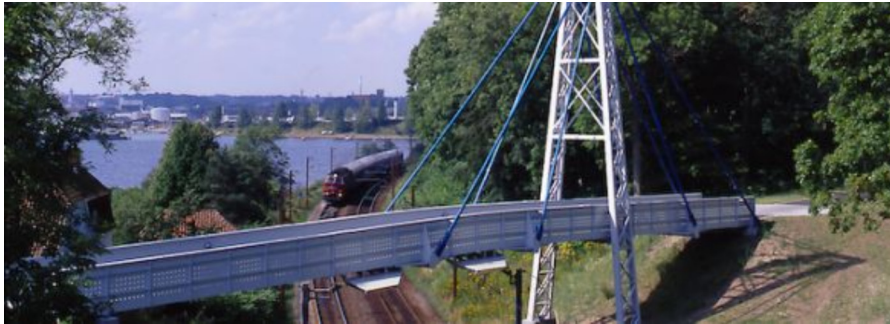
FIGURE 2.25 Plastic bridge reinforced with carbon and glass fibers in Denmark.
