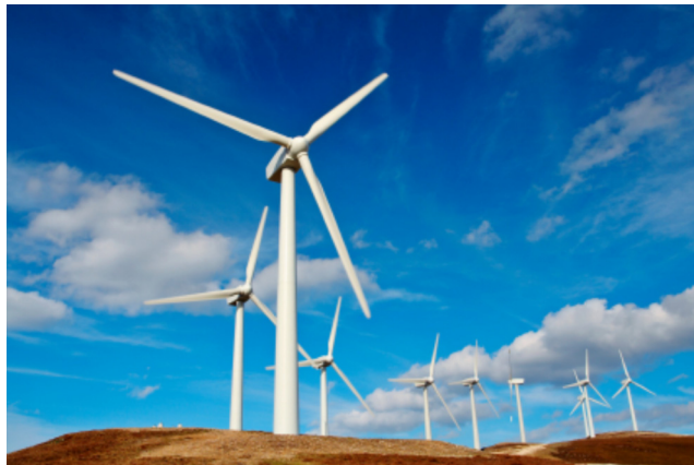
FIGURE 2.26 Wind generator with blades manufactured from composites.
