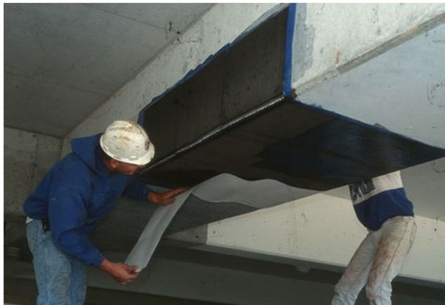
FIGURE 2.24 Reinforcement of concrete columns through the use of fiber composites.
