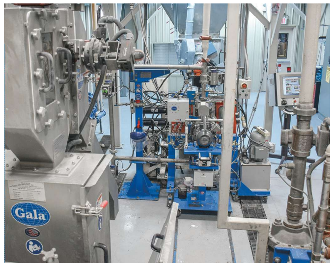
The Primex Color, Compounding & Additives plant in New Jersey houses eight extrusion lines and focuses on high-value, short runs in a variety of materials for a wide range of applications.
