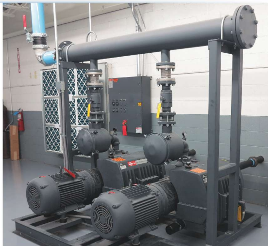
Located in a separate room, two R 5 rotary-vane vacuum pumps from Busch currently deliver vacuum to 23 injection machines at Mar-Bal, with capacity to add up to 10 more presses.
