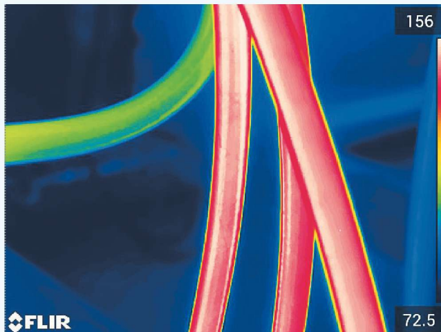
Water lines that are not flowing can be identified quickly using thermal infrared cameras. The greenish-looking line is blocked or turned off.
