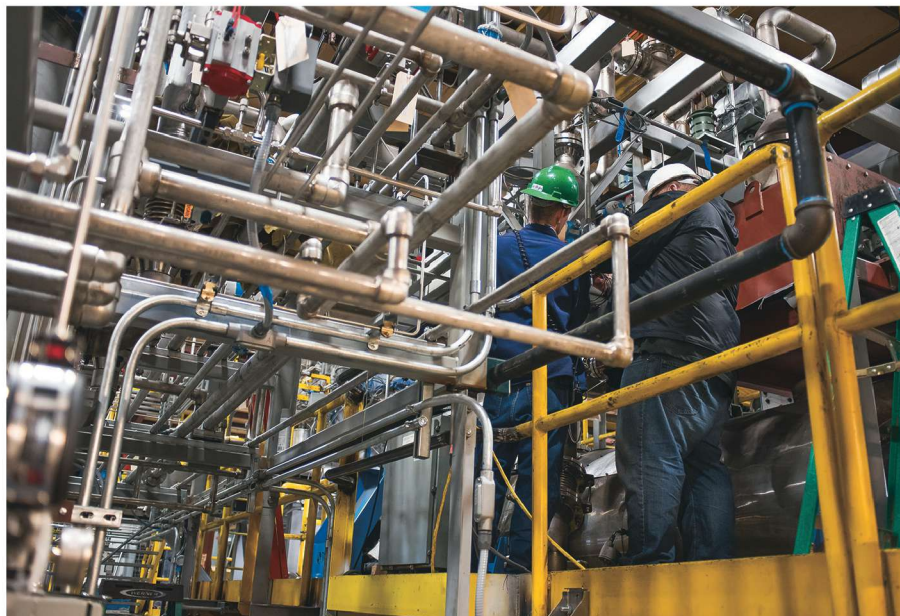
Agilyx retrofitted parts of the Tigard facility originally set up for mixed waste and the plastic-to-oil process to instead perform PS-to-styrene-monomer production.
