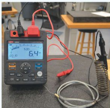
The IR tester shows a heater being tested at 500VDC with an outcome of a perfectly acceptable 6.4 mega-ohms.
