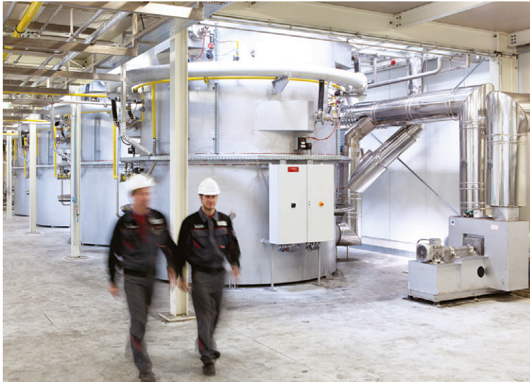
Above: Internal view of the Pyrolyx tyres-to-carbon black production plant at Stegelitz in Germany
