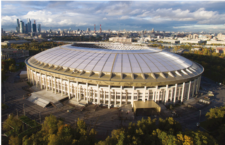
Above: Covestro is selling off all its polycarbonate sheet assets - such as those used in the Luzhniki Olympic Stadium in Russia
