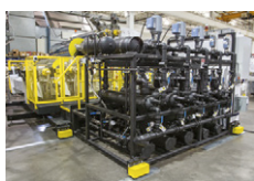
5 Zone Temp Station
