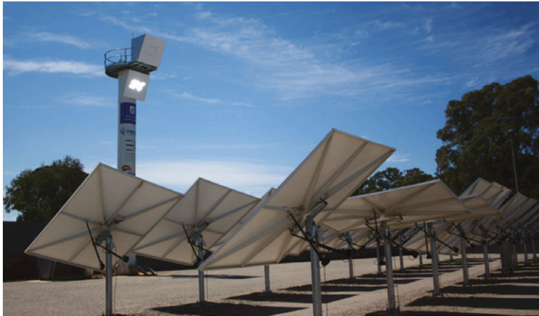
Above: Australian researchers are developing solar energy heliostats that use plastics instead of glass
