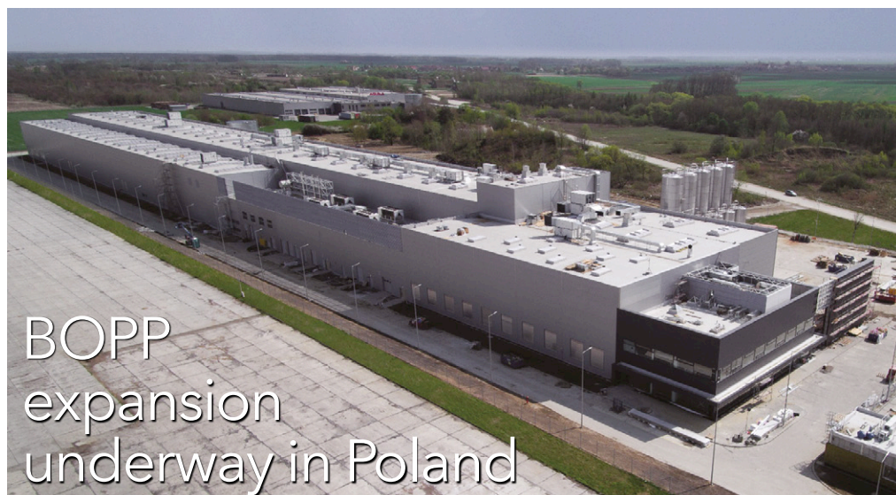
The new plant has an annual BOPP film capacity of 40,000 tonnes
