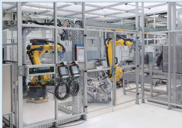
6 BETAFORCE polyurethane adhesive is robotically applied for bonded attachments and then cured in a short oven cycle.
