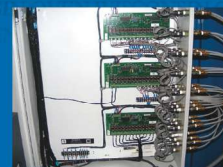
Pressure Transducer Monitoring Lines
