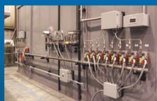
Vacuum Piping System w/ Pressure Transducer & Thermocouple Jack Panel
