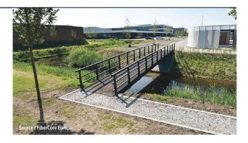
compared to traditional materials are its high strength, low energy requirement during construction, low maintenance requirement and long service life, with no rot or corrosion. As a result, the bridge material is expected to last for at least 100 years.
