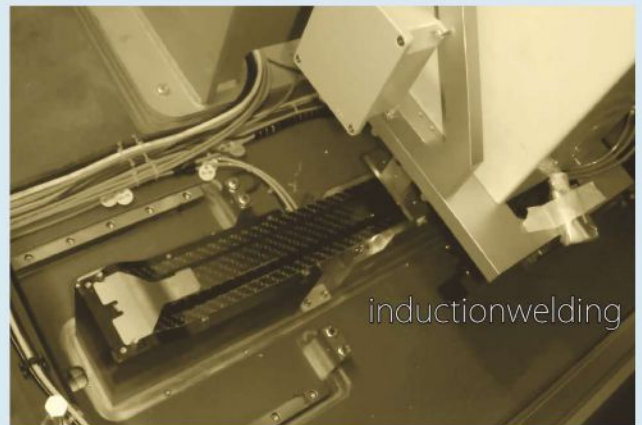
6 The robot then places clamping units on the three brackets, after which the induction joining unit lowers onto the middle bracket. The induction coil causes the metal bracket to heat up, melting the underlying composite's PA6 matrix.
