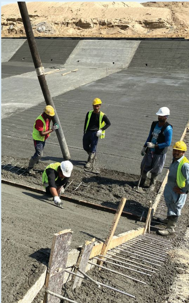
6 Concrete is poured on top of the rebar, then tamped and compressed to remove air bubbles.
