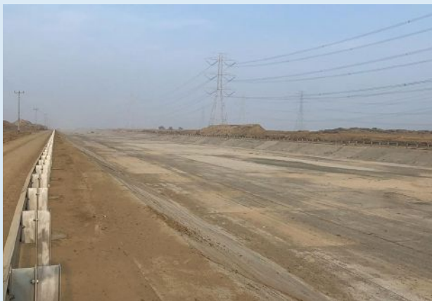
7 The finished reinforced concrete channel in Jizan will direct flood water away from roads and industrial production facilities.
