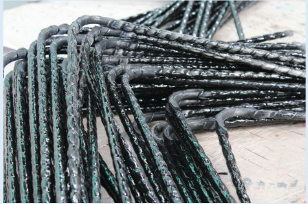
4 Straight and bent GFRP rebar is shipped to the construction site.
