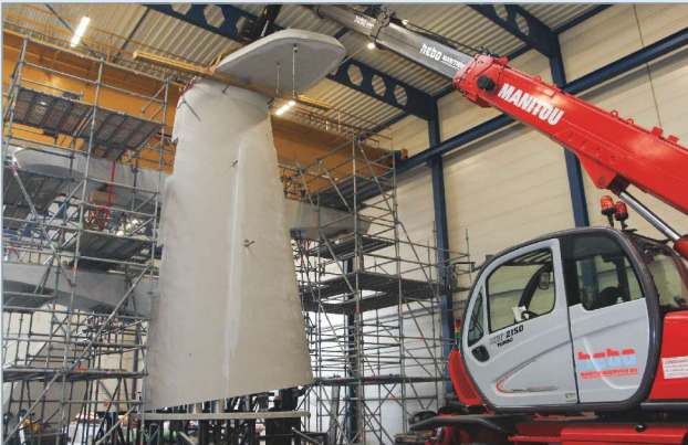
8 Each leg was lifted by crane onto a rail-mounted fixture and slid into scaffolding that located and supported legs and platforms during assembly.
