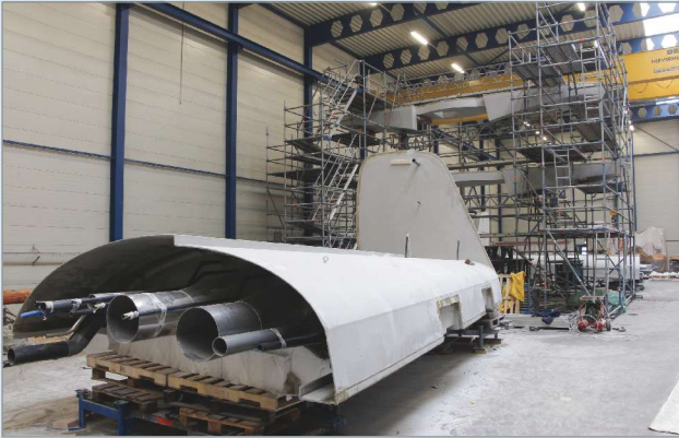
7 The composite legs were prepared for final assembly, inserting exhaust pipes and cable chases.
