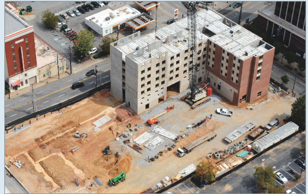
6 After steel angles and plates embedded in each of the precast panels were welded to those in adjacent walls and floors, the building structure in that locale was complete. Source | Aerial Innovations of Georgia / Metromont
