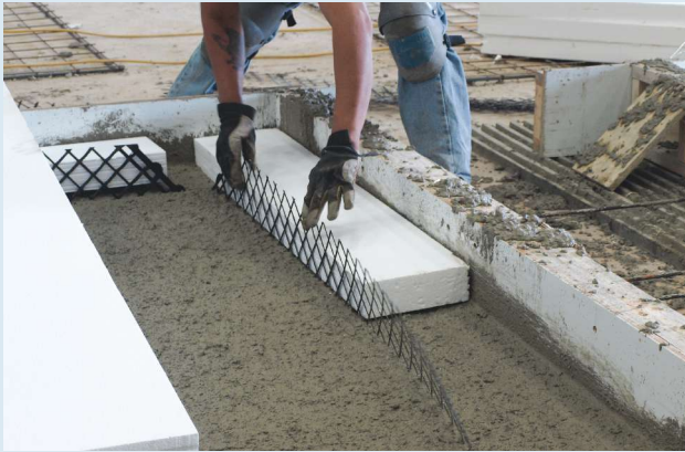
1 EPS foam boards were placed on top of the first concrete pour of the exterior wythe. Source | AltusGroup
