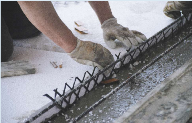
2 C-GRID strips were placed in between the foam boards and pushed down into the wet concrete of the exterior wythe. Source | Metromont
