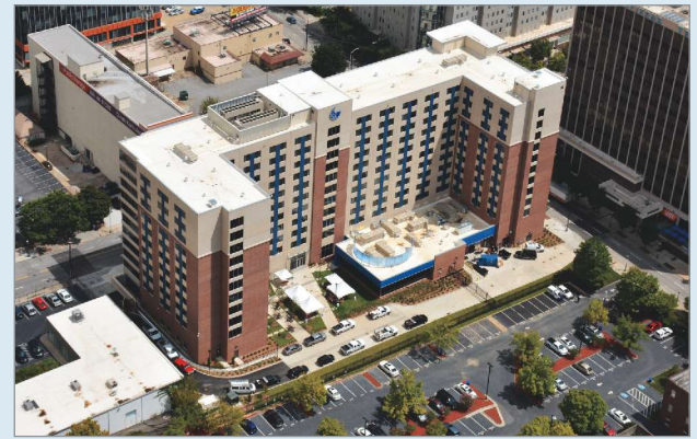
7 As the previous step was completed, building trades could proceed immediately with installation of systems and interior finishes, progressively finishing the building. Source | Aerial Innovations of Georgia / Metromont
