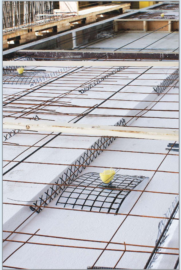
3 Prestressed steel cables and other steel reinforcement were placed on top of the EPS foam prior to the final concrete pour. The yellow objects are inserts for crane lifting points, each anchored with a square of C-GRID. Source | Metromont
