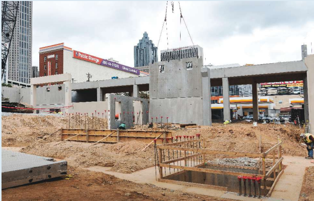
5 Completed wall panels were loaded onto trucks and delivered to the construction site, where they were lifted by a crane and set into place.
