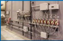
**Vacuum Piping System w/ Pressure Transducer & Thermocouple Jack Panel**
