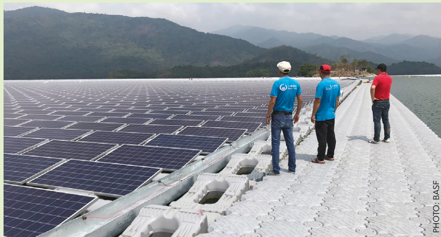
Pontoons for floating solar panel systems in China are blow moulded in HDPE containing light stabilisers from BASF
