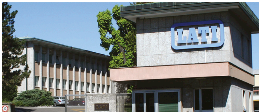
Above: LATI is updating its pilot production plant
