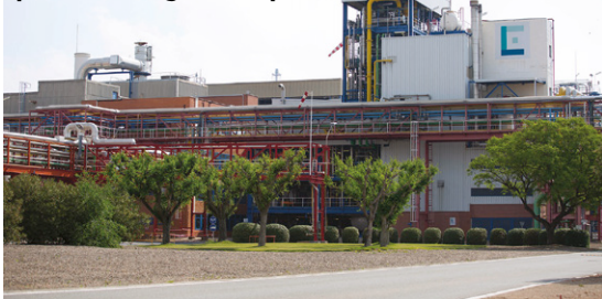
Elix Polymers manufacturing plant at Tarragona in Spain
